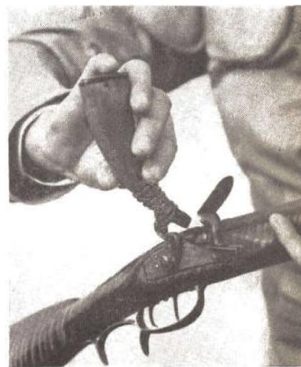
Excess patching removed, patched ball seated on powder charge, priming with fine powder—rifle is ready.
